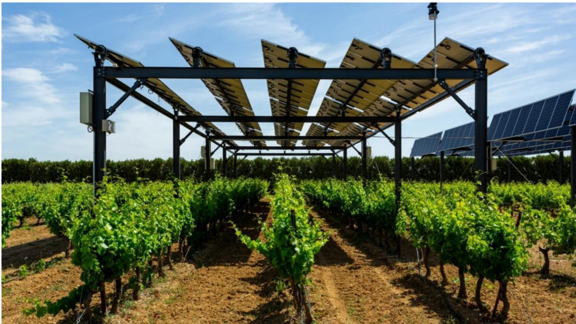
Figure 15. Installation of the "intelligent shading" of the San Gabriel Winery. Source: Laura Cano Liébana, 2022
